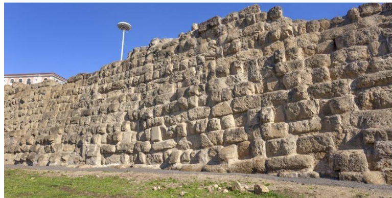
Fig. 3 Cyclopean masonry - The wall attributed to Servius Tullius (578-534 BC)
