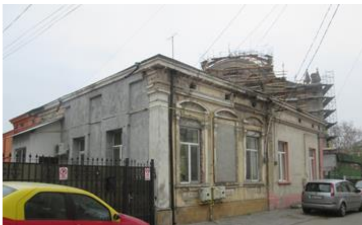
Fig. 18 9 Rubinelor Street – Interventions on historical buildings: modification of window openings by masonry fillings
