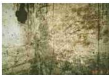
Fig. 12 Mold on the damp wall
