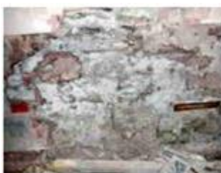
Fig. 13 Mold on drywall
