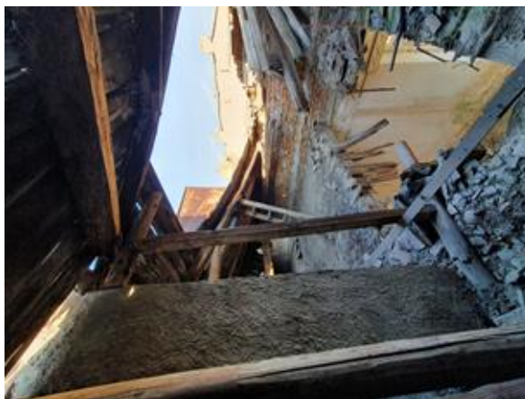
Fig. 20 Building on Mihai Eminescu Street – Collapsed floor
