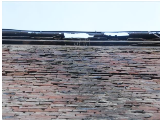
Fig. 2 Moisture due to the penetration of rainwater through degraded gutters
