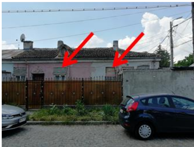
Fig. 17 11.Frumoasă Street – Interventions on historical constructions: modification of window openings by nonwoven masonry fillings
