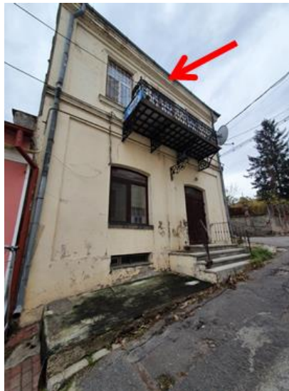
Fig. 1 Moisture due to the penetration of rainwater through degraded gutters
