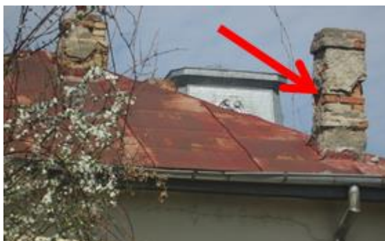
Fig. 14 11 Vapoarelor Street – Weakening of the chimney section
