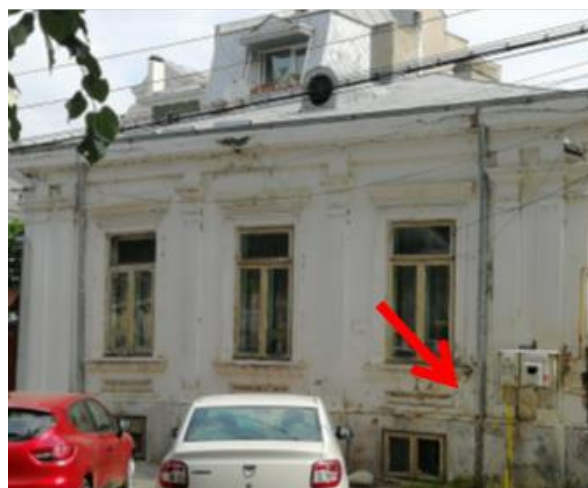
Fig. 3 38 B-dul Al.I.Cuza Street – Grinding effect of plaster due to moisture
