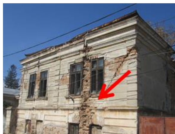
Fig. 4 10 Marăști Street – Degradation of the brick due to the phenomenon of repeated freeze-thaw of stagnant water on the surface of the wall
