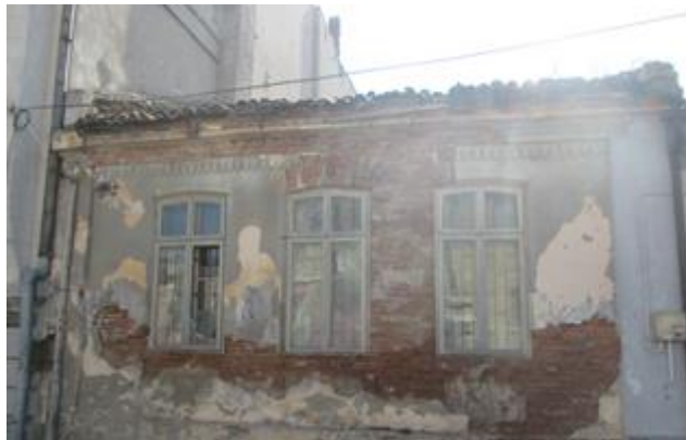
Fig. 5 6 Danube Street - Degradation of the brick due to the phenomenon of repeated freeze-thaw of stagnant water on the surface of the wall
