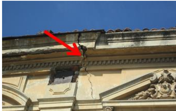
Fig. 15 7 Vapoarelor Street – Inclined crack extended over several asises
