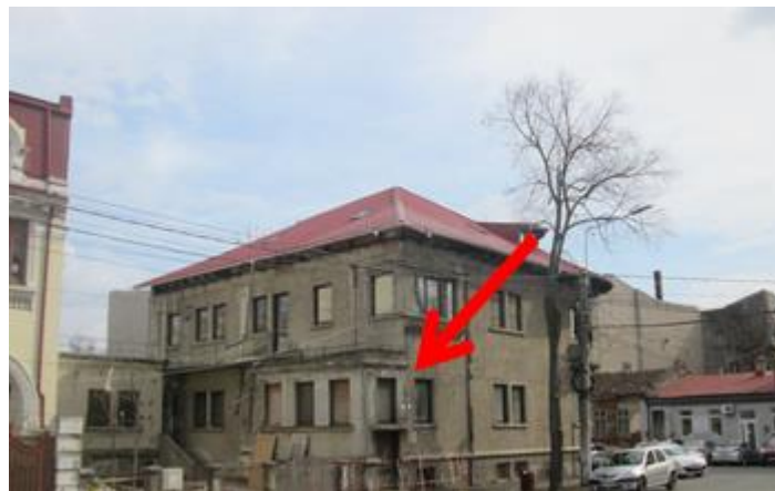
Fig. 16 9 Calea Călărașilor Street – Vertical separation crack
