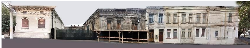
Fig. 4 Streetview with the facades of the buildings no. 5, 3 and 7, C.A. Rosetti Street
