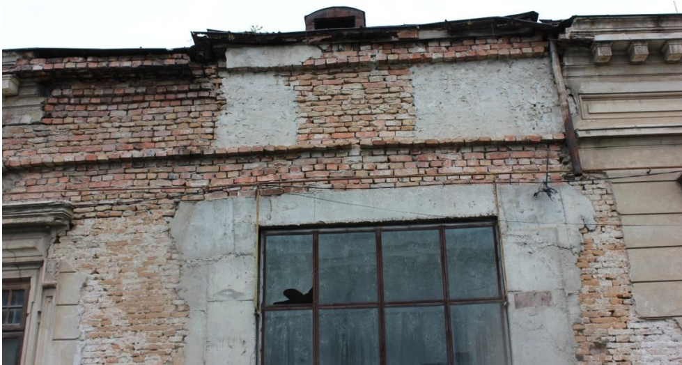
Fig. 16 The elevation stage in the evolution of the building – Entrance façade
