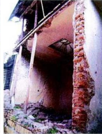
Fig. 3 View of the back façade
