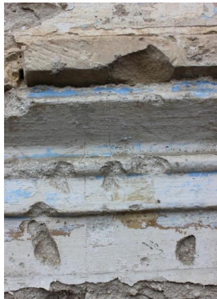
Fig. 15 Layers of the south façade
