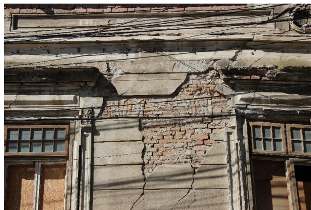
Fig. 17 The closure of the flattened arches – Street façade
