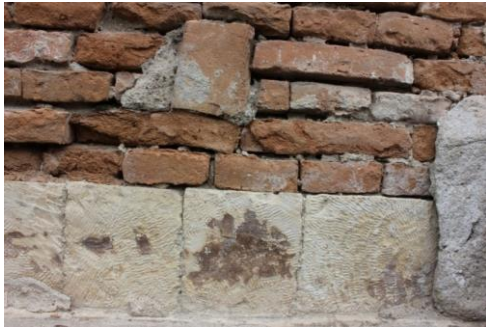
Fig. 12 Traces of processing on garden façade
