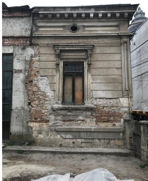
Fig. 5 Detail of the façade intervention in a previous stage
