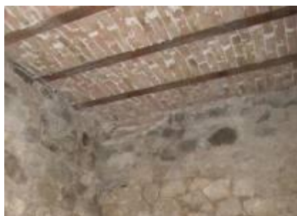
Fig. 1 Floor made of metal beams on which brick vaults discharge [7]
