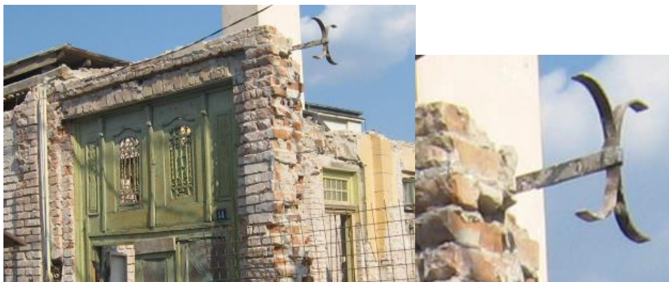
Fig. 16 A detail of tie rod with anchor highlighted in the situation of a building being demolished. Image of building built in the 2nd part of the 19th century in D. Bolintineanu Street, Brăila city
