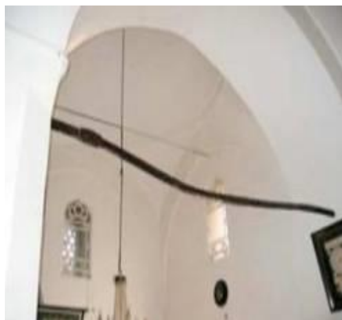
Fig. 6 Tie rod tension and interior of the Atik Ali Pasha Mosque in Istanbul (15th century) [1]
