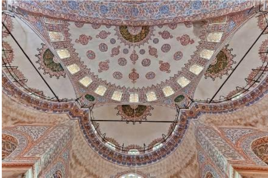
Fig. 3 Metal truss - Blue Mosque in Istanbul (17th century) [11]
