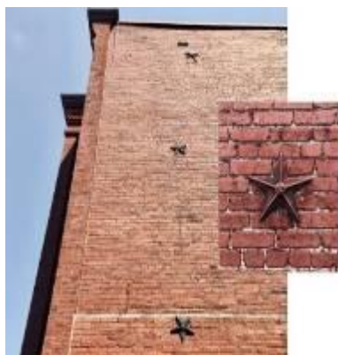
Fig. 9 Star anchor, the anchor plate in the shape of a star with 5 corners – Washington D.C. (U.S.A.) [18]
