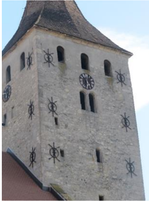
Fig. 10 The position of the tie rods with ornamental anchors at a historical tower, Alba Iulia City
