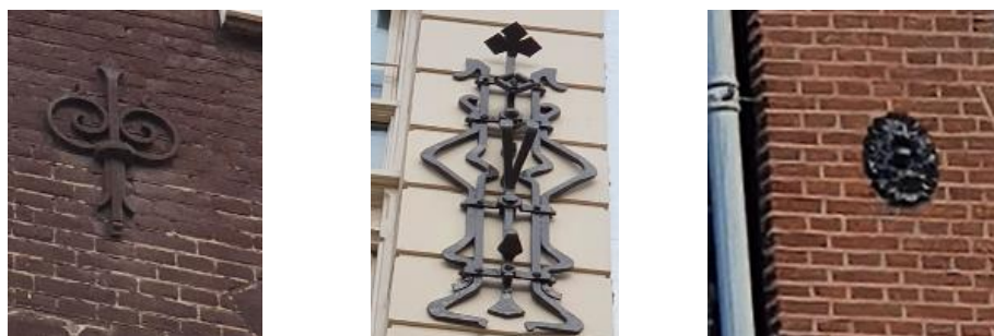
Fig. 13 Anchor types – detail
