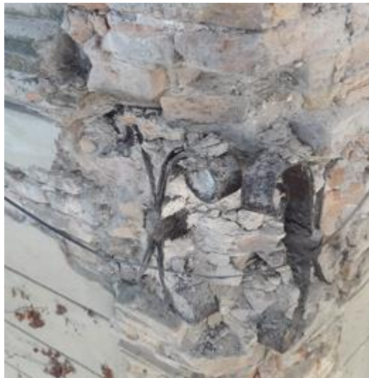
Fig. 15 Tie rod detail at the intersection of the exterior load-bearing walls of the facade
