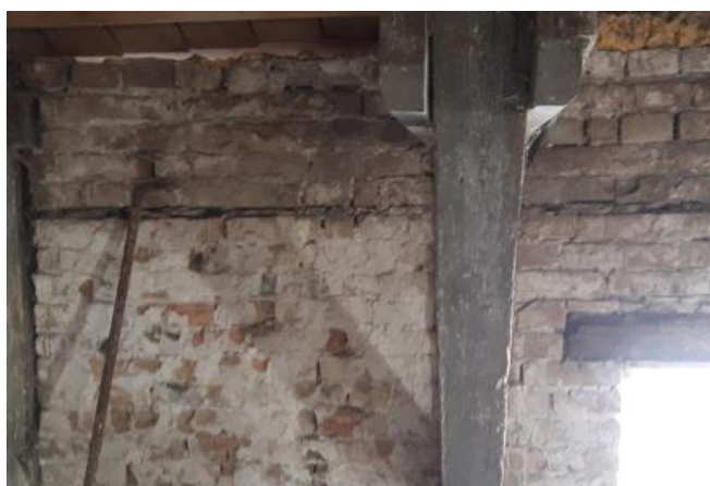
Fig. 18 Anchoring the pediment by means of an inclined plate. Building, Sulmona Street Constanța City
