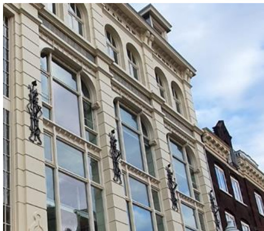
Fig. 12 Multi-storey building with metal anchoring elements next to the floors - Netherlands
