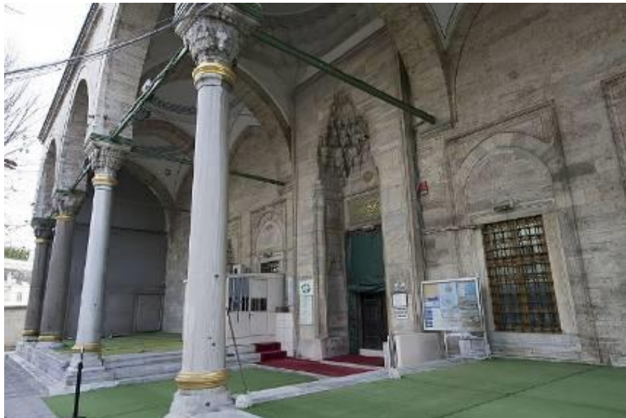
Fig. 4 Iron tie rods at the entrance of the Atik Ali Pasha Mosque Istanbul (15th century) [12]
