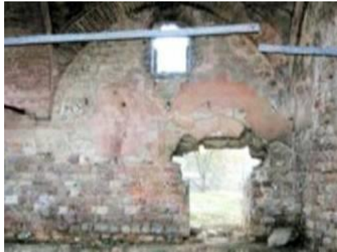
Fig. 7 Tie rod yielding in the central area, the Palace Edirne - kitchen building (15th century) [1]
