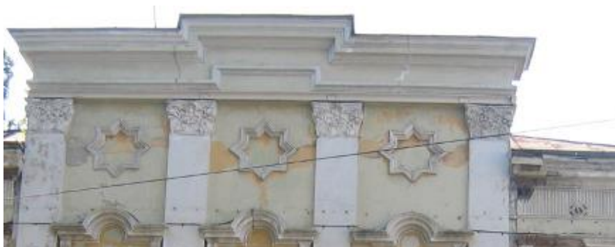
Fig. 22 Anchoring the pediment, at the level of the bridge, to the frame with the creation of ornaments in the shape of an eight-pointed star on the facade of a memorial house in Brăila
