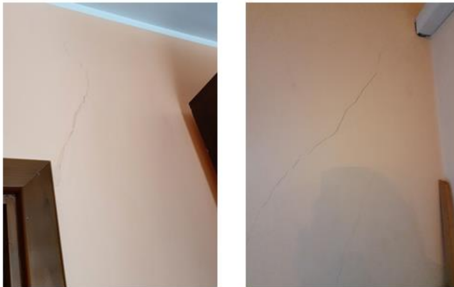
Fig. 5 and Fig. 6 Cracks in a block of large panels, Galati [3]
