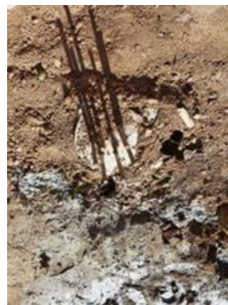
Fig. 5 Detail of micro-piles
