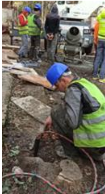
Fig. 15 Injection through sleeve tubes of the soil, Source: Mădălina Iordache
