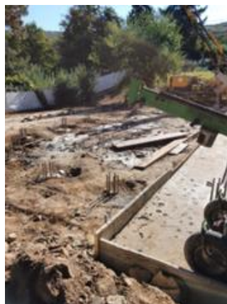
Fig. 4 Micro-piles in the new altar area, lateral façade
