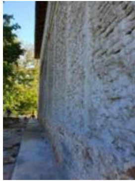
Fig. 8 Area for injection with stable suspension of bentonite and cement Source: Mădălina Iordache
