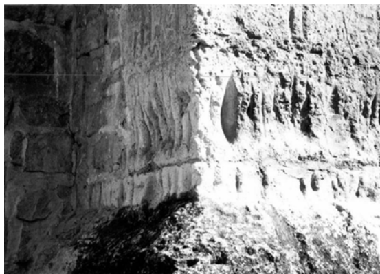
Fig. 2. Degradation of limestone blocks vertically layed
