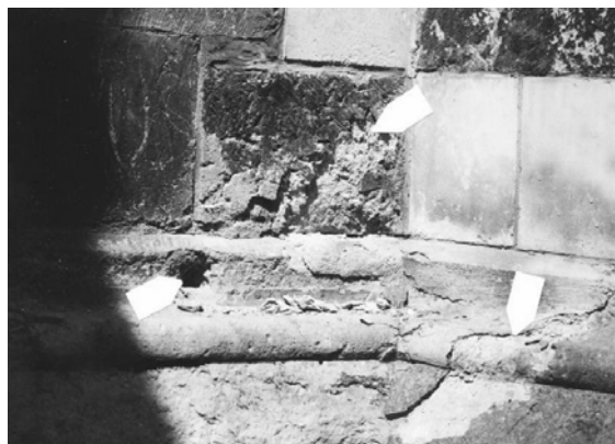
Fig.4. Limestone with small diameter pores – massive dislocations from rock mass, at Saint Michael Cathedral, Cluj-Napoca
