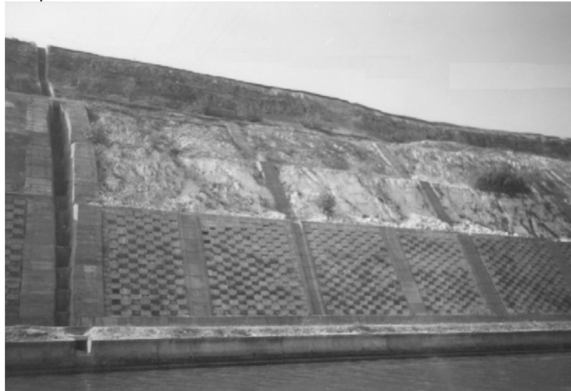
Fig.8. Bank slope of limes protected with prefab caissons
