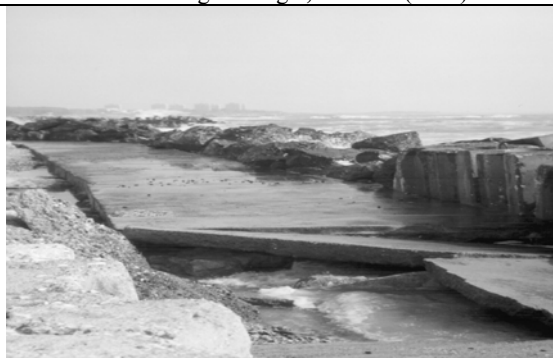
Photo. No. 1 Top of groin collapsed (groin 3, Jupiter – 08.08.2002)
