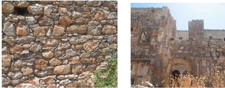
Fig. 10. Masonry restored and being restored using existing components
