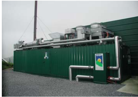
Fig. 10. Container of the gas engine
