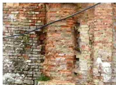
Fig. 8. The effect of grinding brick masonry caused by repeated freeze-thaw phenomenon of stagnant water wall surface
