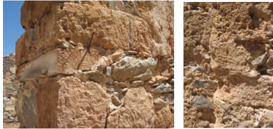
Fig. 7. Details on stone degradation due to moisture
