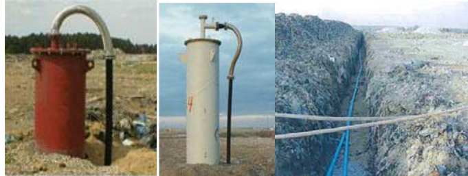
Fig. 4 – Example of wells drilling and degassing trenches
