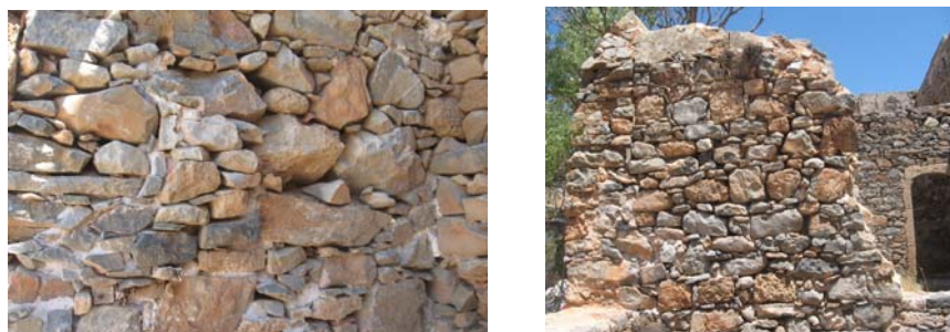
Fig. 2. Dry stone masonry (without mortar)
