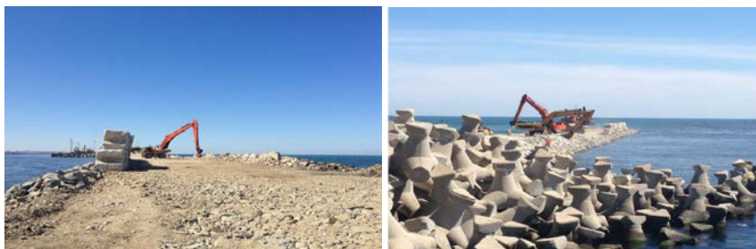
Fig. 3. Works on the North Breakwater [15]
